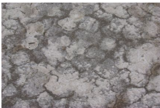
Figure 2 Shows a close up of the soil and scald at chainage 225m. In January 2000 this soil was underwater for 3 months.
